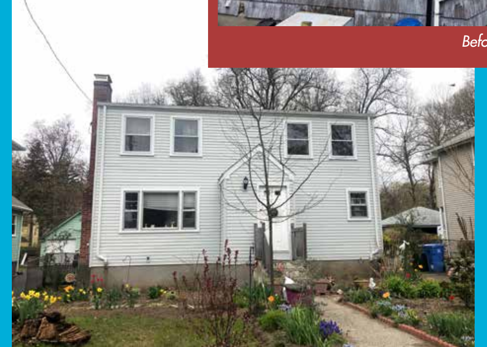
After the restoration of the veteran home in Hartford, in partnership with Rebuilding Together
